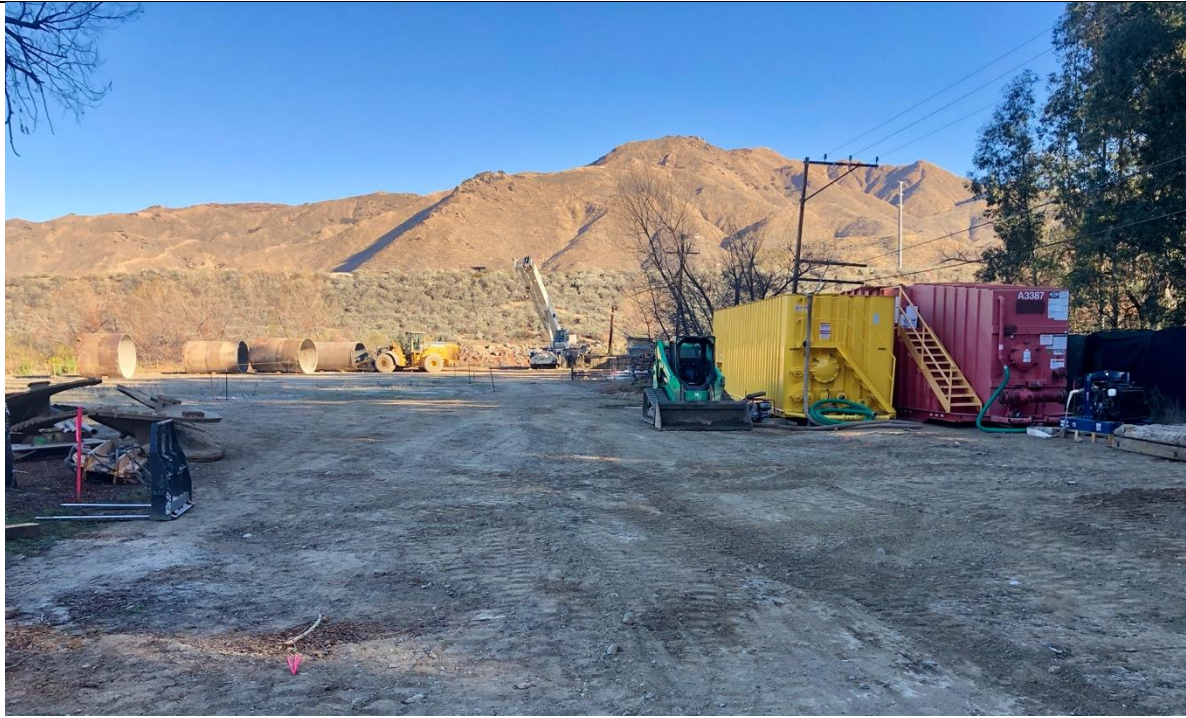
Photo 5 – Staging area between TSPs 520 and 522. Photo facing east
