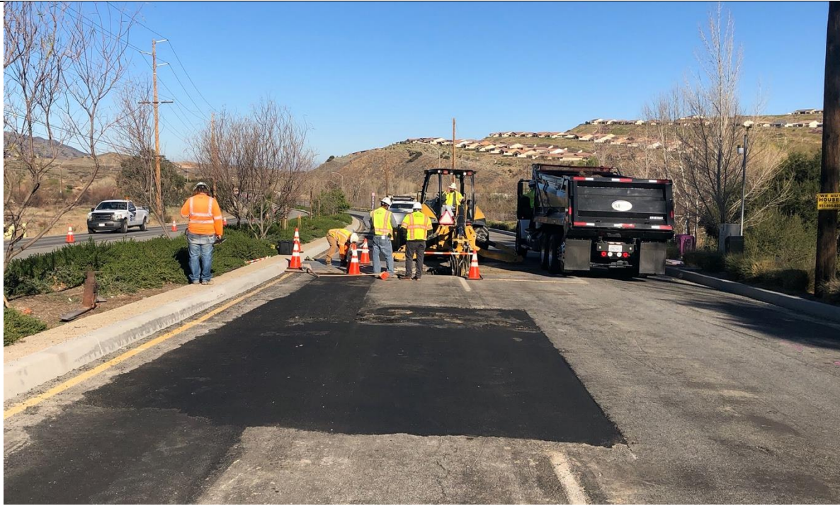
Photo 7 – Segment 8 underground installation within Temescal Canyon Road. Photo facing north
